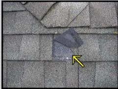
General condition appeared serviceable with the exception of the following item(s): One damaged or missing shingle was visible on the roof. We recommend repair or replacement of this shingle to prevent moisture intrusion.
