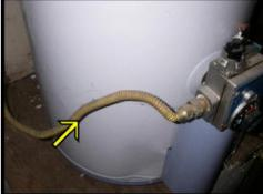
Pressure relief valve was noted, not tested. A water shutoff valve was installed. The unit is plumbed with a flexible brass type gas line. These type of lines have been known to deteriorate over time and are no longer used. We recommend upgrading the gas line to the unit for safety enhancement.
