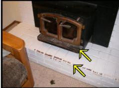
There did not appear to be a minimum of 16" from the burn area / door to combustible materials. The hearth should extend a minimum of 16 inches in front of the firebox / door. This is typical in several jurisdiction's. We recommend researching the county building requirements prior to the release of the inspection contingency. This is a fire / safety hazard. Correction is recommended.
