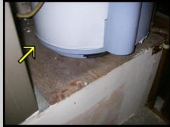
The general condition appears serviceable with the exception of the following item(s) listed below. The floor of the water heater compartment appeared to be sagging. This can be caused by the weight of the unit or a moisture condition. We recommend repair or replacement.
