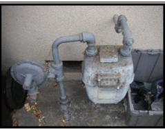
Gas meter was located on the left side of the home. We recommend the installation of a gas meter shut off wrench at the meter so the gas can be turned off in the case of an emergency.
