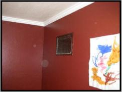
Return air register noted in the kitchen. This is an improper installation. We recommend moving the return air register to an open central area of the home to ensure proper air flow back to the furnace.
