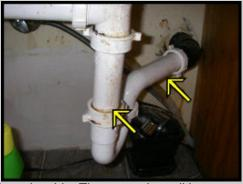
Faucet appeared serviceable. The general condition appeared serviceable at the time of the inspection with the exception of the following item(s) listed below. Waste plumbing below the sink was leaking. We recommend repair to the drain line.
