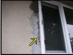
The walls are clad with stucco which ends below the soil level. Current standards call for stucco to end above the level of the soil. This helps deter pests and moisture wicking. Upgrades are recommended.
