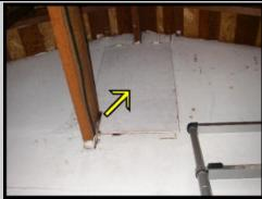
Walls of the garage were not fully visible due to stored items. The door to the attic from the garage was made of combustible materials. This is a potential safety hazard. We recommend installing a door to the crawlspace which is fire rated.
