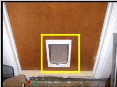
Self closer was functioning properly. General condition appeared serviceable with the exception of the following item(s): Pet door penetrates through the door. This compromises the fire rating of the door. This is a safety hazard. Correction is recommended. No threshold was noted at the interior garage door. We recommend installing a threshold to prevent unwanted pests from entering.
