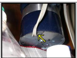
General condition appeared serviceable with the exception of the following item(s): Clamp was missing on the wire below the garbage disposal. This is a potential safety hazard. Correction is recommended.
