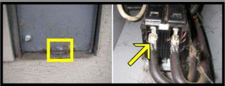
Grounding system is present. General condition appeared serviceable with the exception of the following item(s): The dead front cover is a type which does not have screws to keep the dead front cover in place. This can be a safety hazard for children who could open the panel. We recommend the installation of a lock or screws which will make the removal of the dead front cover difficult for children.
