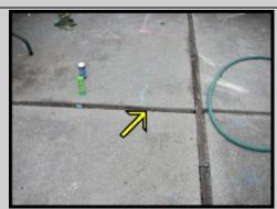
Common cracks were noted on the patio. We recommend sealing the cracks to prevent further erosion.
